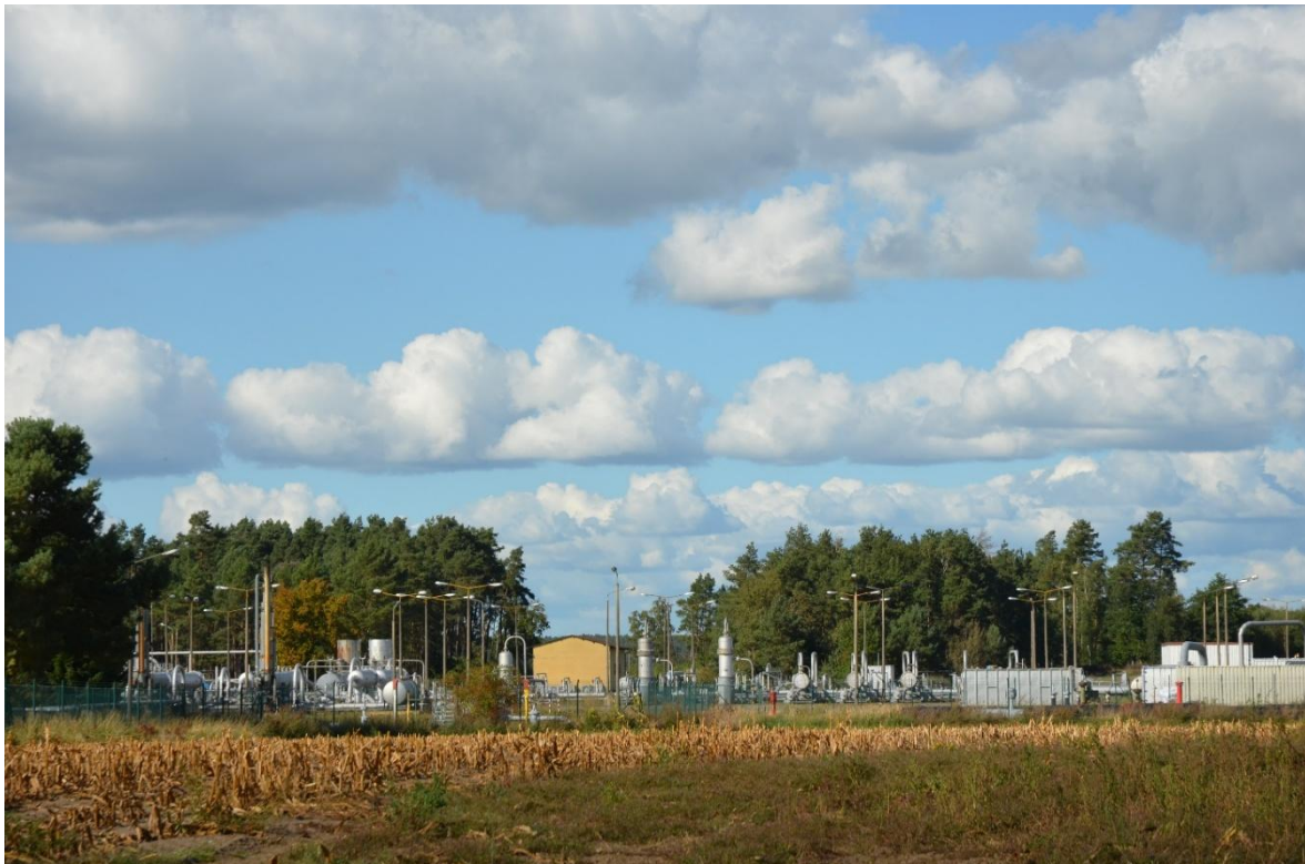
Figures 2 and 3: Prof. Dr Petra Schneider, Hochschule Magdeburg-Stendal. Direct lithium extraction (DLE) at an existing natural-gas production site. Neptune Energy's pilot plant at Steinitz (Altmark) is testing the extraction of lithium from formation brine produced during natural-gas production.
