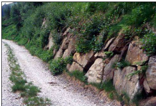
Block stone wall planted with green alder after 7 years
