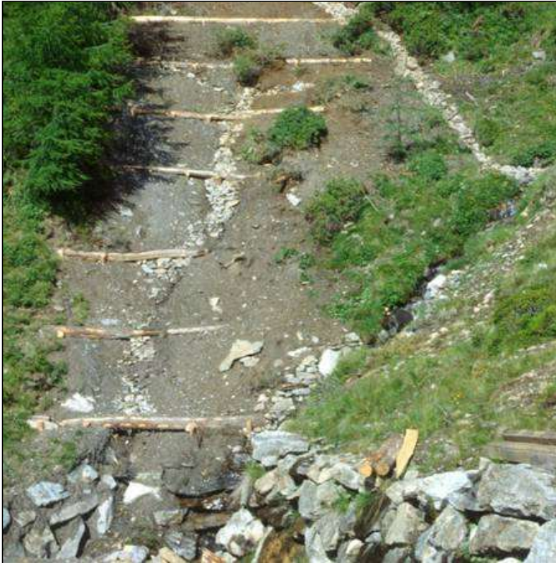
Drain pipe covered with stones
