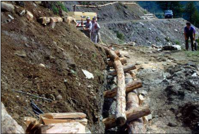
Simple live crib wall, just built
