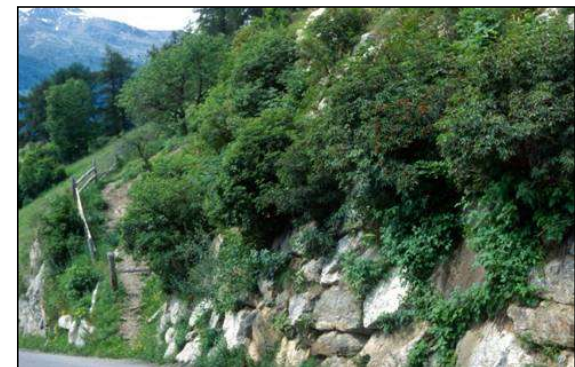
Block stone wall planted with various hardwoods after 6 years
