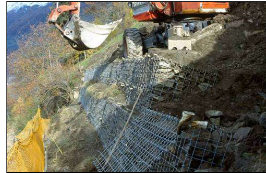
Construction of Gabions
