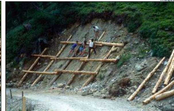
Securing with living hanging grate
