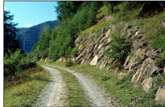
Block stone wall planted with hydroseeding after 17 years
