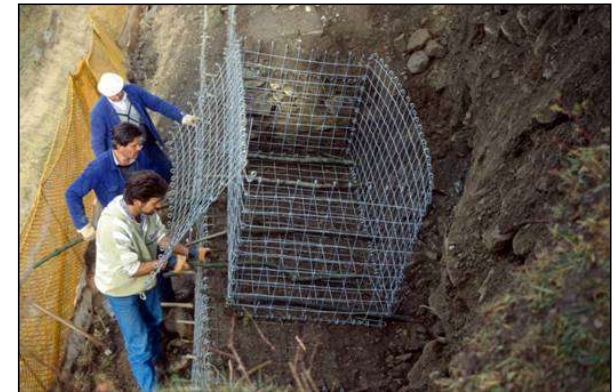
Insert the willow cuttings through the galvanized grid down to the natural soil
